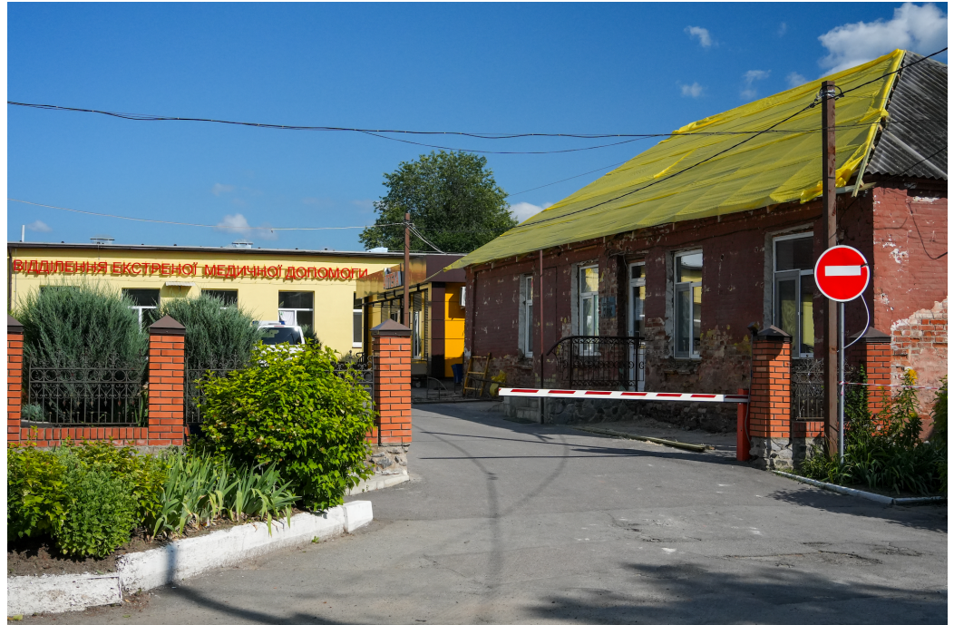
A medical clinic in Dergachy under construction after damage from Russian forces.
