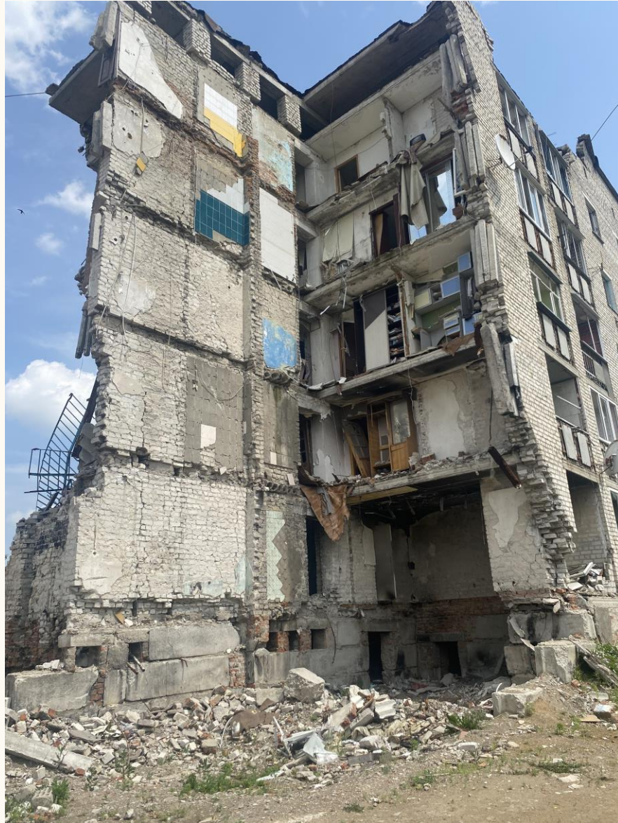
The bombed-out remains of a 40-apartment building at 2 Pershotravneva Street in Izyum.
